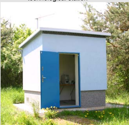
One of the monitoring stations
