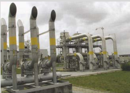
The underground gas reservoir technological station
