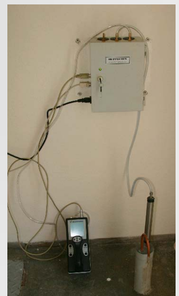
ECOPROBE 5 with a monitoring box comprising switching valves for zeroing, back-up power supply and GSM cellular data communicator.
